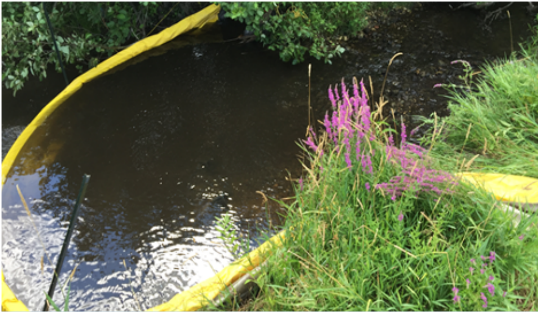
Secured silt curtain holding the current.
