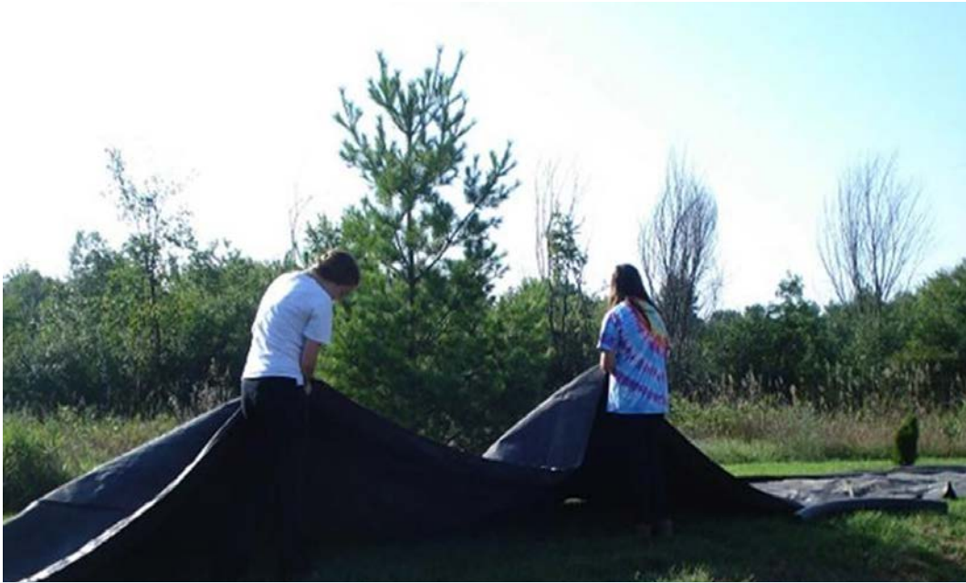
Adding the floats and chains to a silt curtain.
