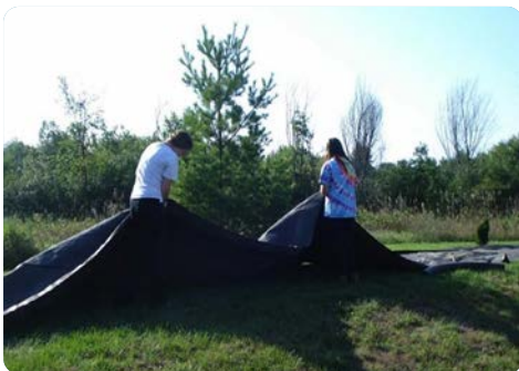
Adding the floats and chains to a new silt curtain.
