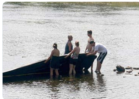
Installing the silt curtain around the work site.
