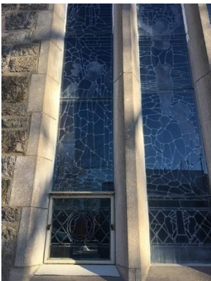
A pretty fresh air inlet that is also stained glass -St. Lambert United Church, Saint-Lambert, QC
