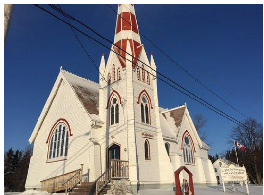
A pretty exhaust chimney, that is also a steeple -St John the Evangelist United Church, Crapaud PEI
