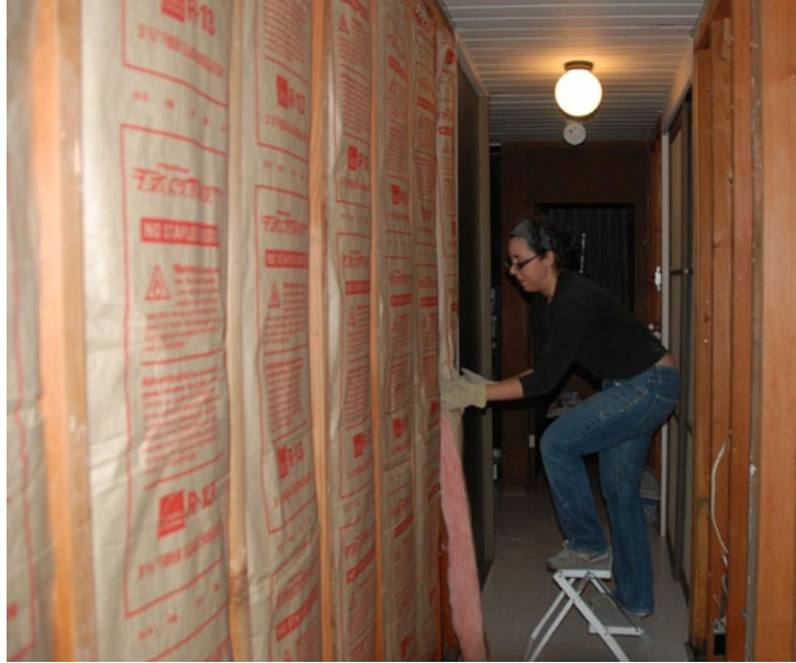
INSTALLING INSULATION. PHOTO CREDIT: NICK NGUYEN, CREATIVE COMMONS
