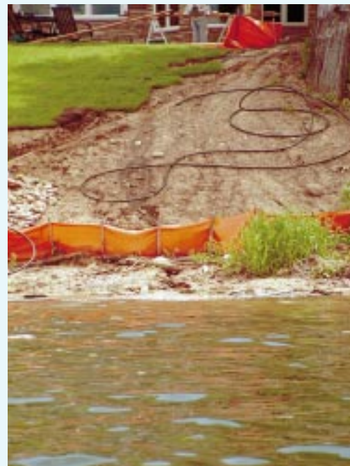
Properly maintained silt fences can minimize erosion caused by construction activities.
