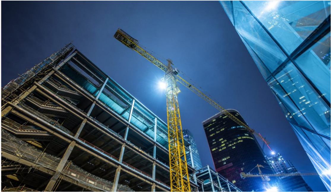
The light from ongoing construction can disrupt species' feeding or breeding behaviours.
